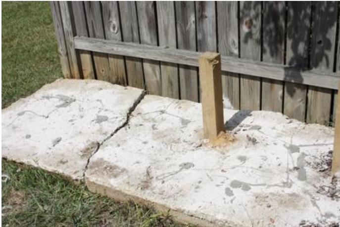
*Here's the slab w/ all holes filled. I covered with plastic and let it cure for 24 hours.*
