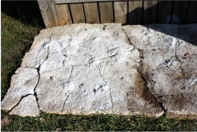
*After 24 hours, the slab was webbed with cracks.*
