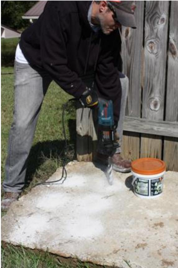
*I used a rotary hammer to drill holes for the Ecobust.*
